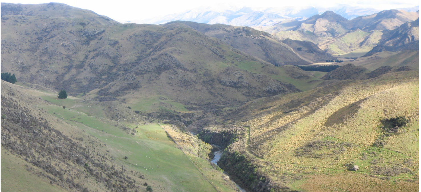
View of the Waitohi River above Seven Hills site. Water level would be within the gorge.
